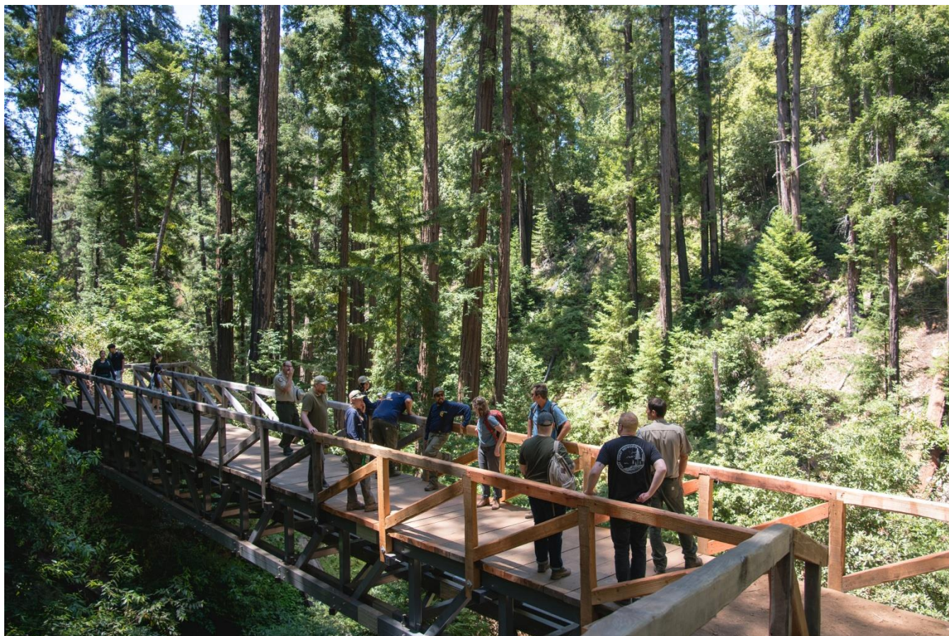
The newly built pedestrian bridge along Pfeiffer Falls Trail in Pfeiffer Big Sur State Park. Photo from Lisa Morales Winner, courtesy of Save the Redwoods League
