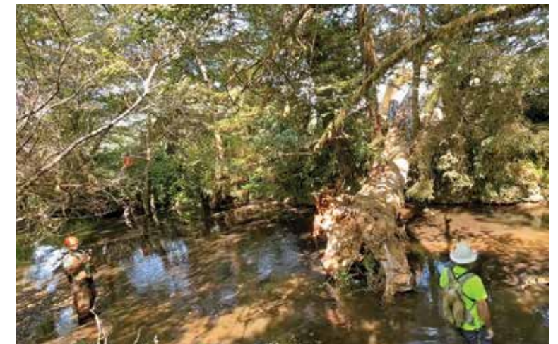
The Yurok Tribe Construction Corporation and Fisheries Department installed large pieces of wood in stream channels to improve habitat for salmon and other aquatic species.
